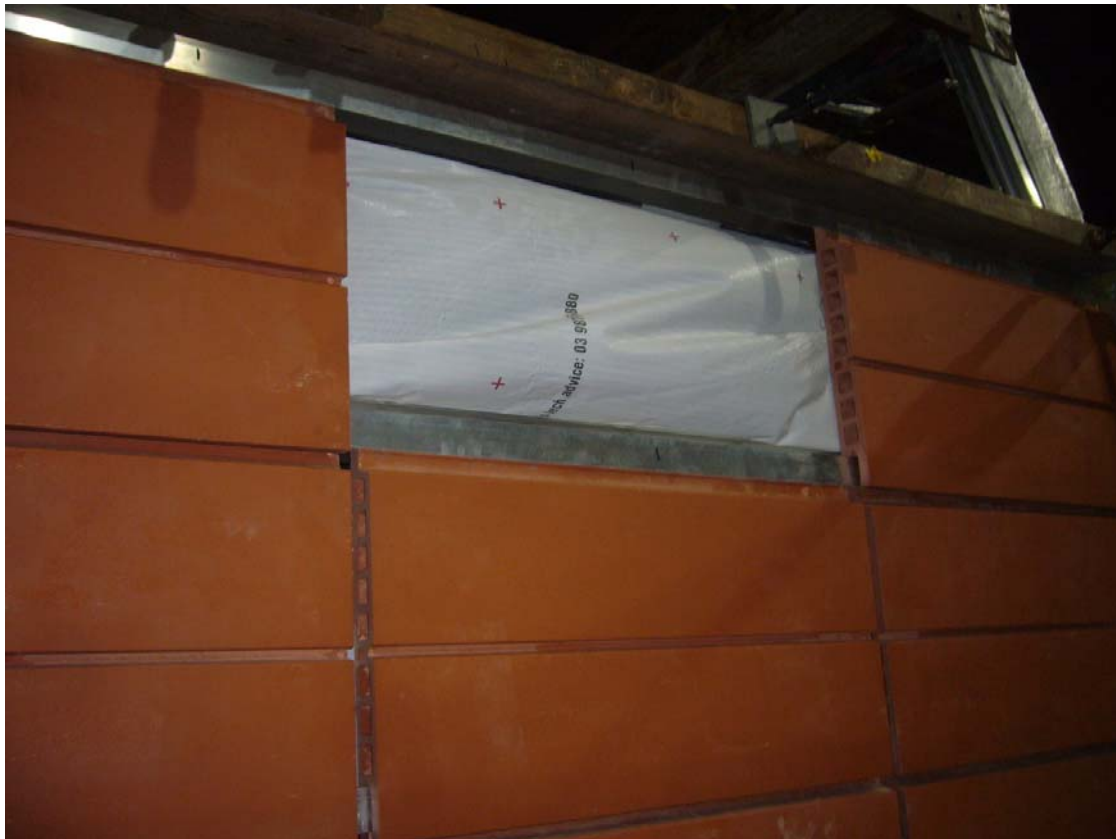
Figure 3: Photograph of the tile to the right of the tile that released.
