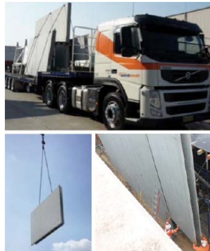
Figure 1.6 – Double Wall Installation Process
