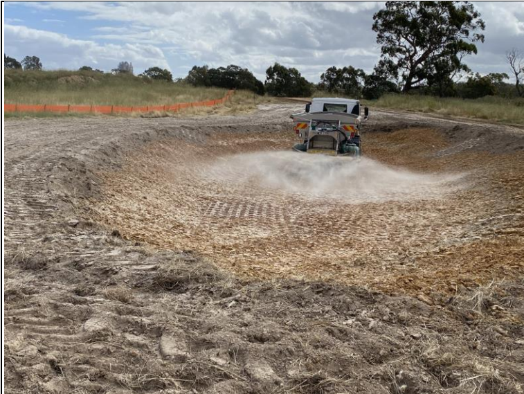
Plate 5 Spreading Gypsum across Completed Dam 10 Source: Austral Bricks Date: 11/12/2020
