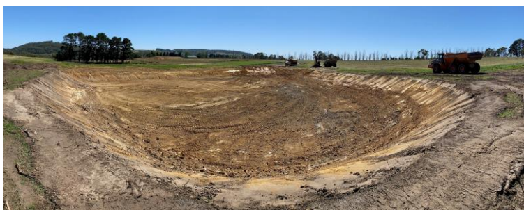
Plate 4 Dam 7 Construction – In Progress Source: Austral Bricks Date: 14/01/2021
