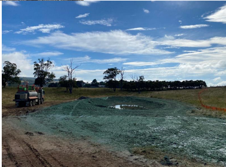
Plate 6 Hydromulch Applied to Completed Dam 10 Source: Austral Bricks Date: 17/12/2021
