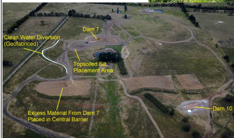
Plate 3 Oblique Aerial of Key Construction Works Source: Austral Bricks Date: 15/12/2021
