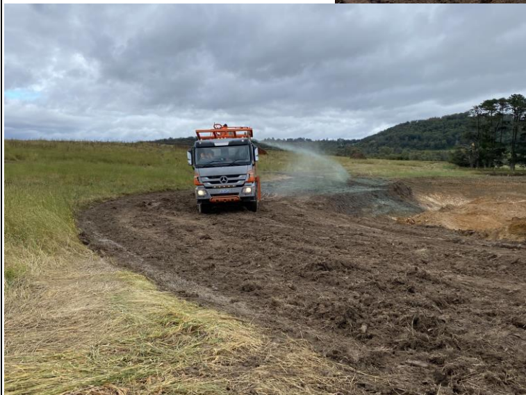
Plate 7 Hydromulching Completed Section of Dam 7 Source: Austral Bricks Date: 22/12/2020
