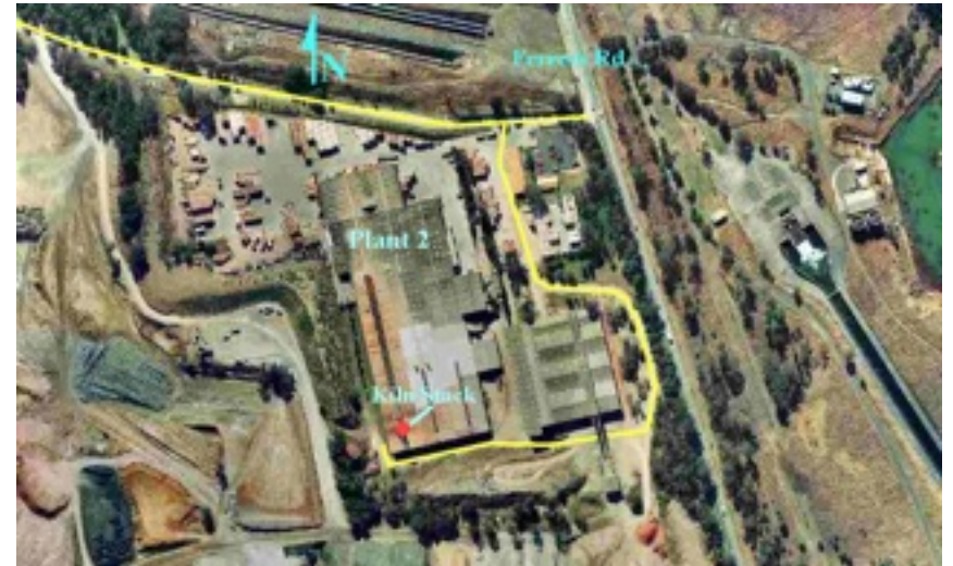
Horsley Park Plant 2
