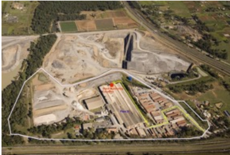
Horsley Park Plant 1
