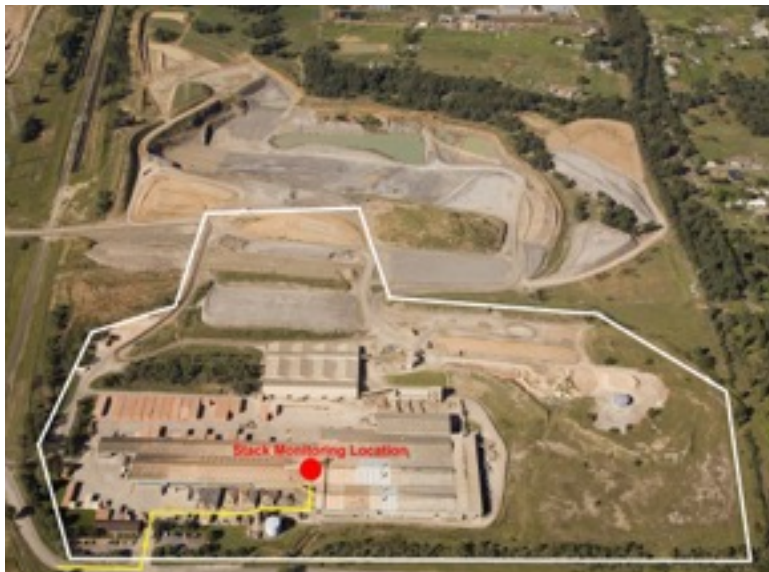
Horsley Park Plant 3
