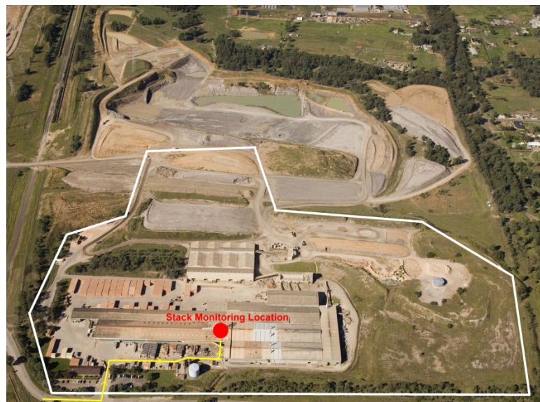
Horsley Park Plant 3
