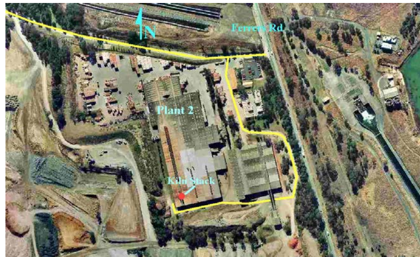
Horsley Park Plant 2
