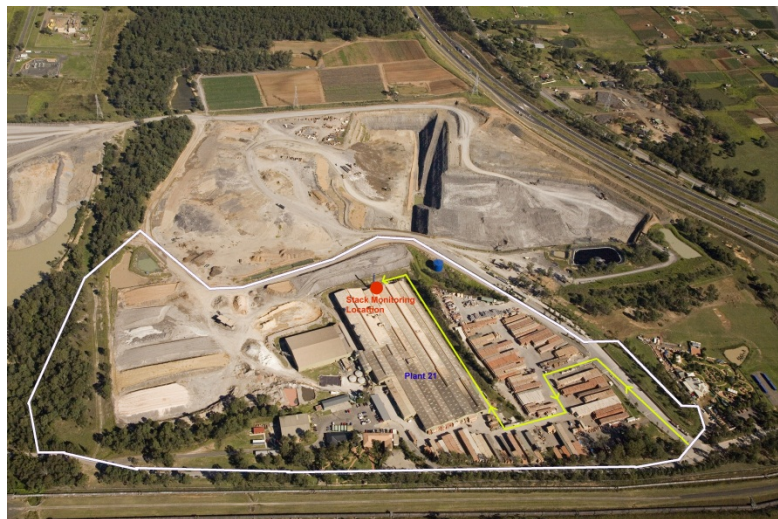
Horsley Park Plant 1
