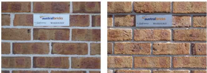
(b) The effect of mortar joint style on the same brick - flush joint and raked joint respectively
