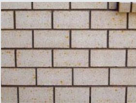
Iron Staining on Brick Faces
