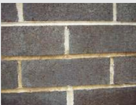
Iron Staining in Mortar Joints
