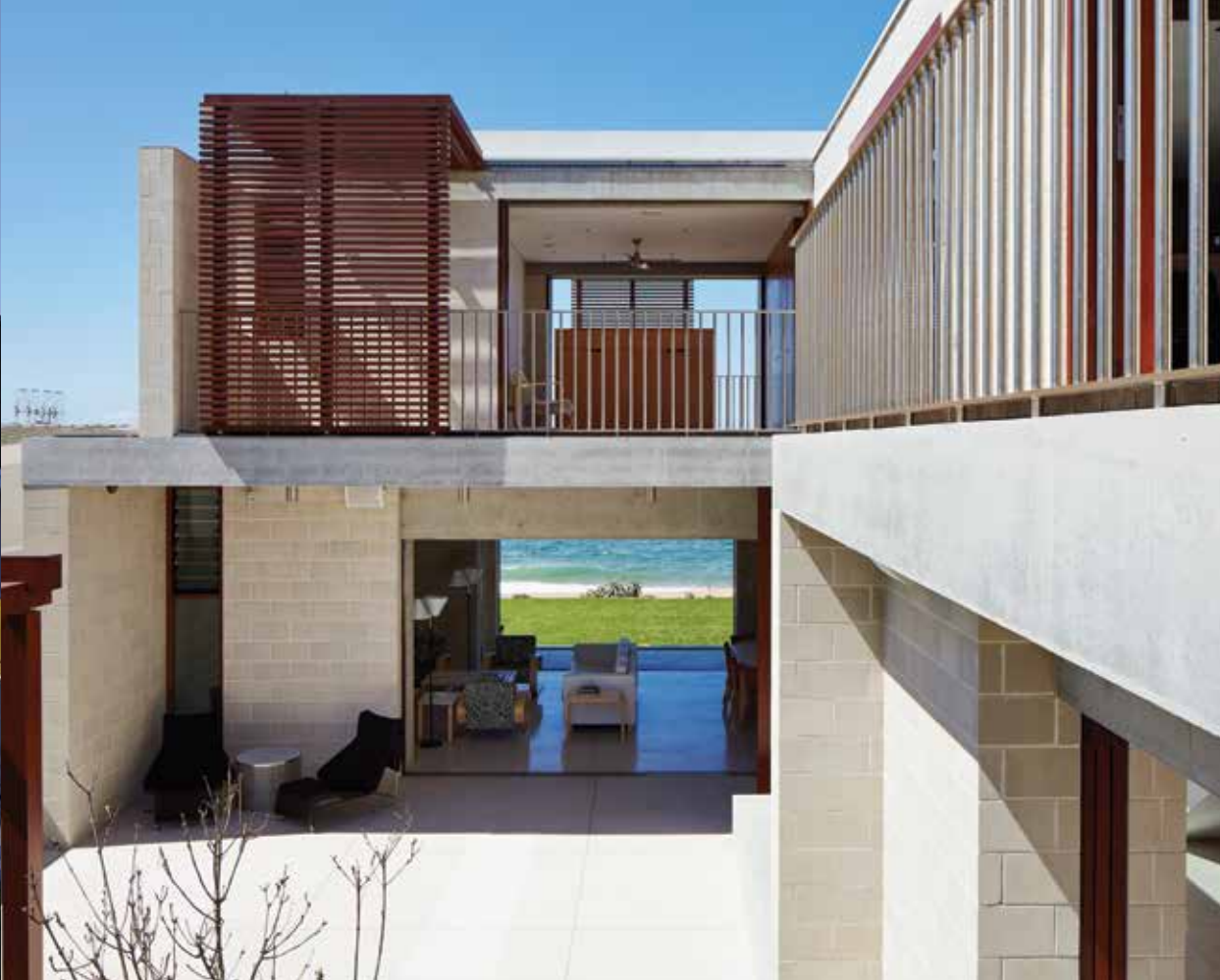
clockwise from bottom left. Concrete masonry is a durable, low-maintenance material in this saline and abrasive environment. The house is set over two levels with living below and sleeping quarters above. The courtyard does double duty, allowing northern light while screening the afternoon wind.
