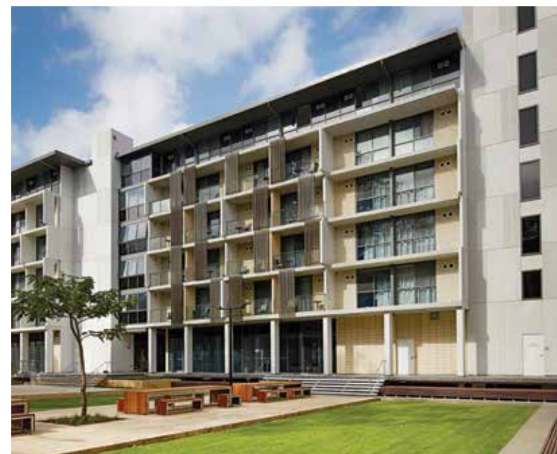
Project: University Hall Location: Thomas Street, Crawley WA Function: Student accommodation Owner: University of Western Australia Architect: HASSELL Structural engineer: Robert Bird Group Builder: Probuild Photography: Douglas Mark Black
