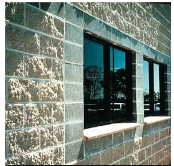
"Angled splitting" to concrete blocks
