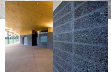
Polished reconstructed granite blocks used for the external skin of a house
