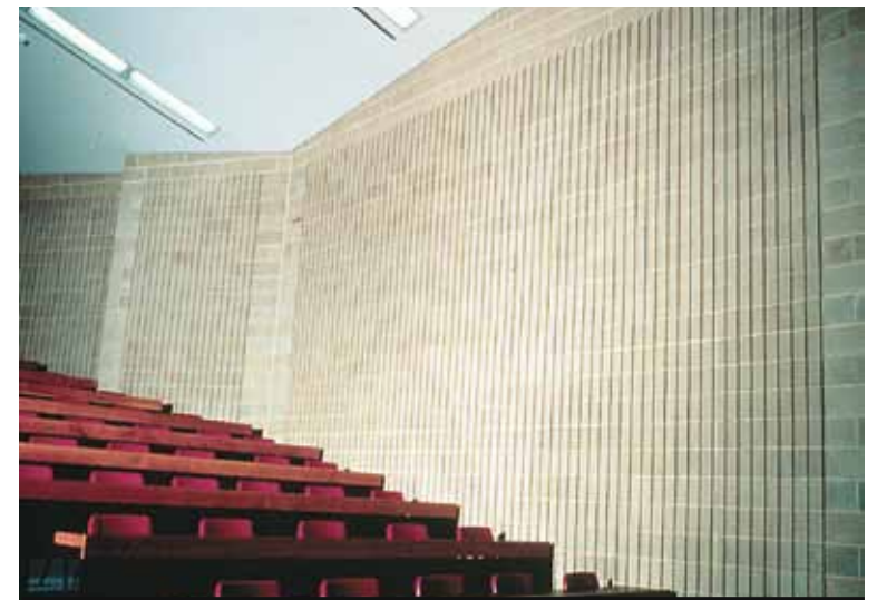
Plain ribbed blocks used to assist acoustics in an auditorium
