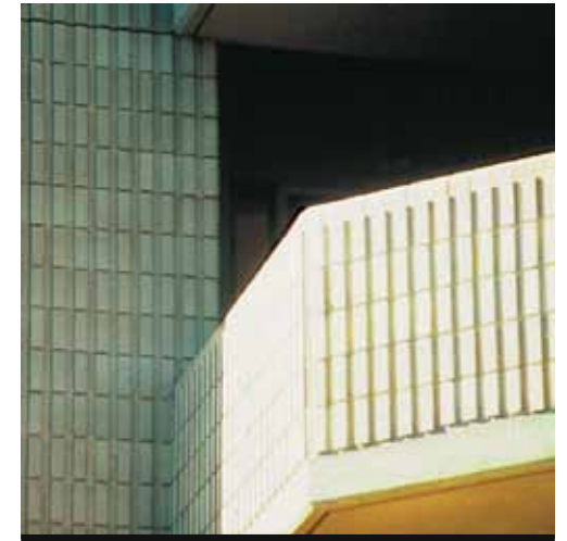
Plain ribbed block to wall and balustrade of residential units
