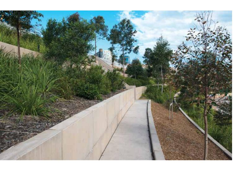
At each stage the Magnumstone blocks, which are hollow, can be filled with aggregate to increase their weight and thus their retaining capacity. When the wall reaches its design height, it can be finished with top units (full or half height).
