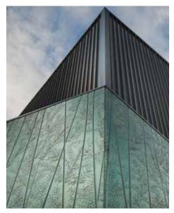
Above: The Nepean Mental Health Centre walls are finished in an engraved bamboo pattern and coloured using Austral Precast's PermaTint system.
