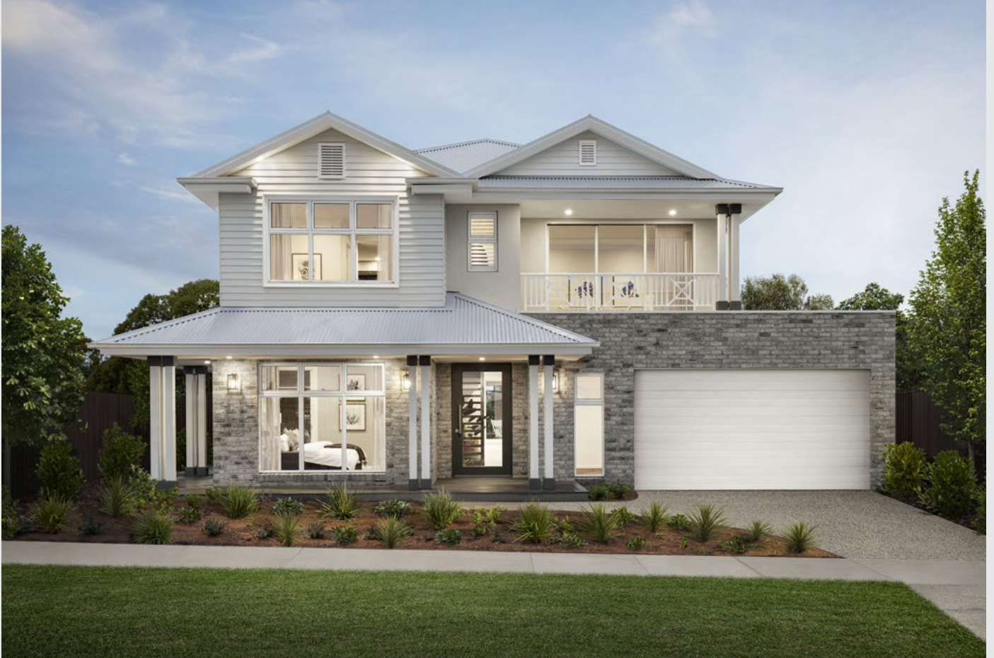
Builder Beachwood Homes
