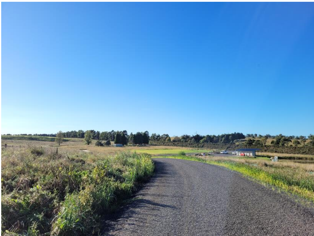
Photo 4 – All major site access roads and associated catch drains are now spray sealed.
