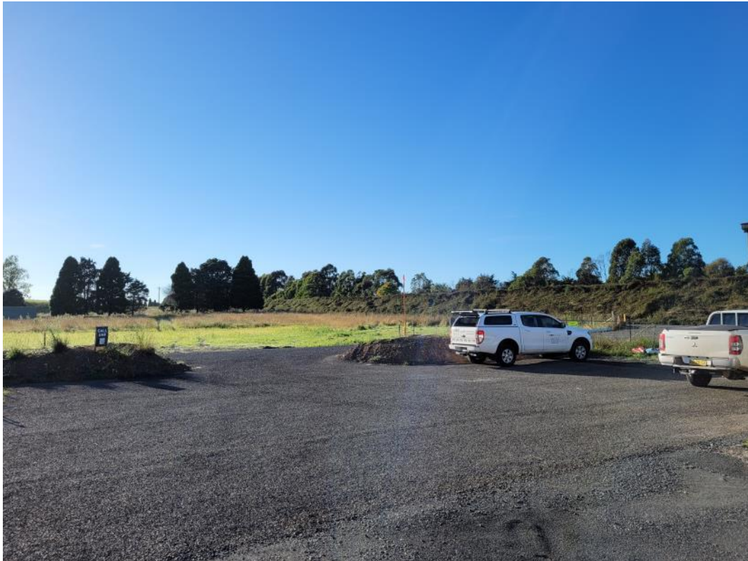
Photo 3 – Site compound surface has been stabilised. Laydown area and amenity barriers have also been stabilised (i.e. hydromulched) and has achieved at least 70% ground cover.
