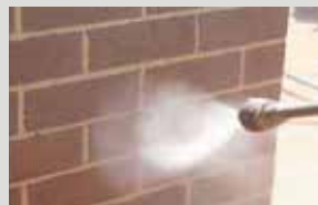
CORRECT HIGH PRESSURE CLEANING <7000 kPa, >15°, >500 mm
