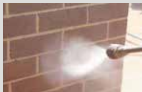
CORRECT HIGH PRESSURE CLEANING <7000 kPa, >15°, >500 mm
