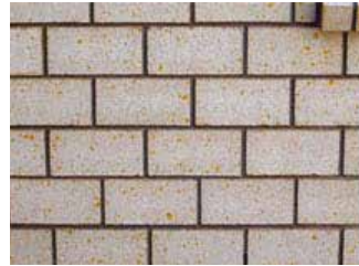
Iron Staining on Brick Faces
