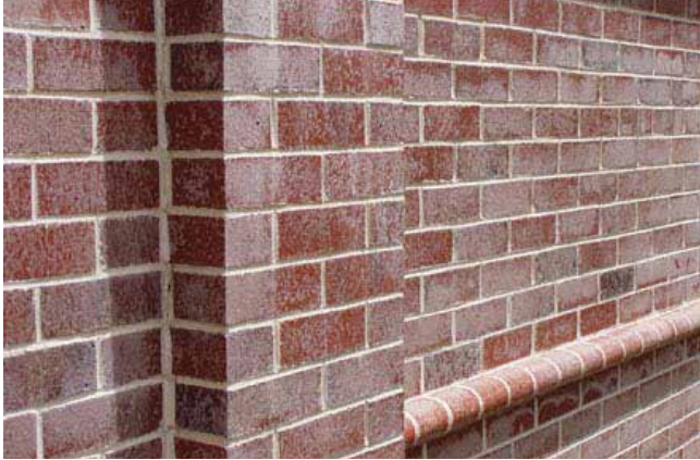
Iron Staining on Brick Faces
