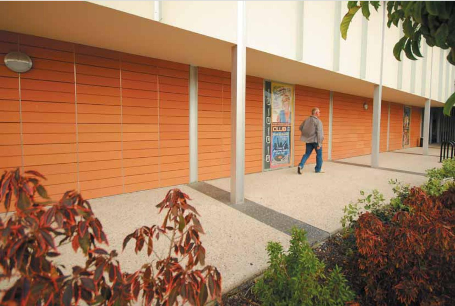
Because Terraçade tiles are made from kiln fired terracotta, the colours are permanent. Additionally every tile is further protected with Terrashield, a factory applied surface treatment that allows the easy removal of stains, spills and grime. With normal maintenance, Terrashield-protected tiles can be expected to have similar wear characteristics and last as long as ceramic glazed tiles.
