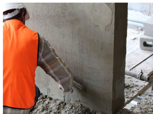
Step 2: Under Coat (a)
