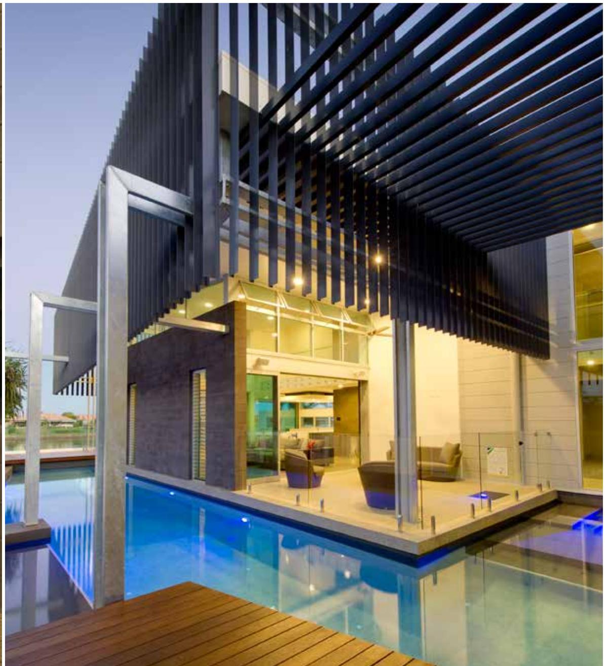
Austral Masonry GB Smooth masonry in Pewter is used in the spine walls that run along both storeys through the main breezeway of the house. The masonry is located internally and externally to maximise thermal mass – an essential component of an energy efficient design – and to maintain a visual flow between the indoor and outdoor areas.
