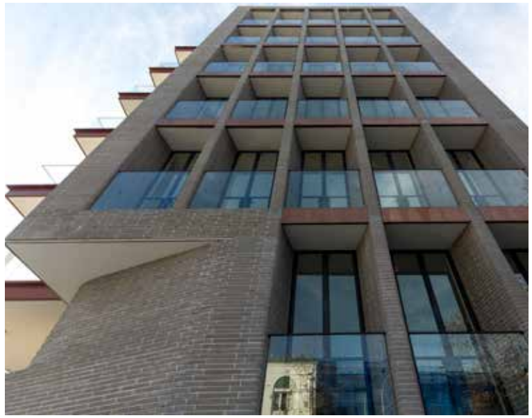
Bullnose masonry units used on front elevation
