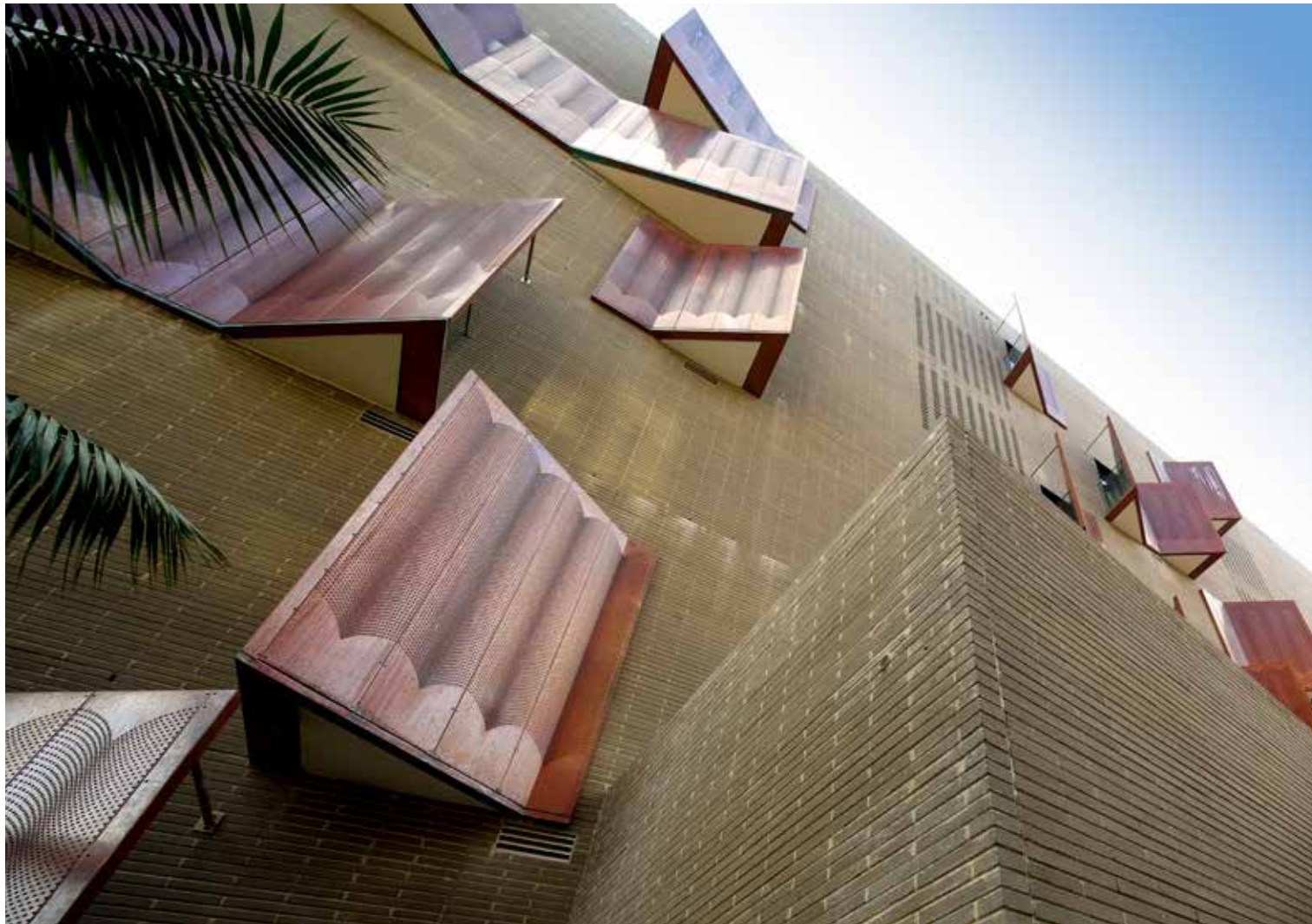
Breeze walls create a striking feature and improve thermal performance
