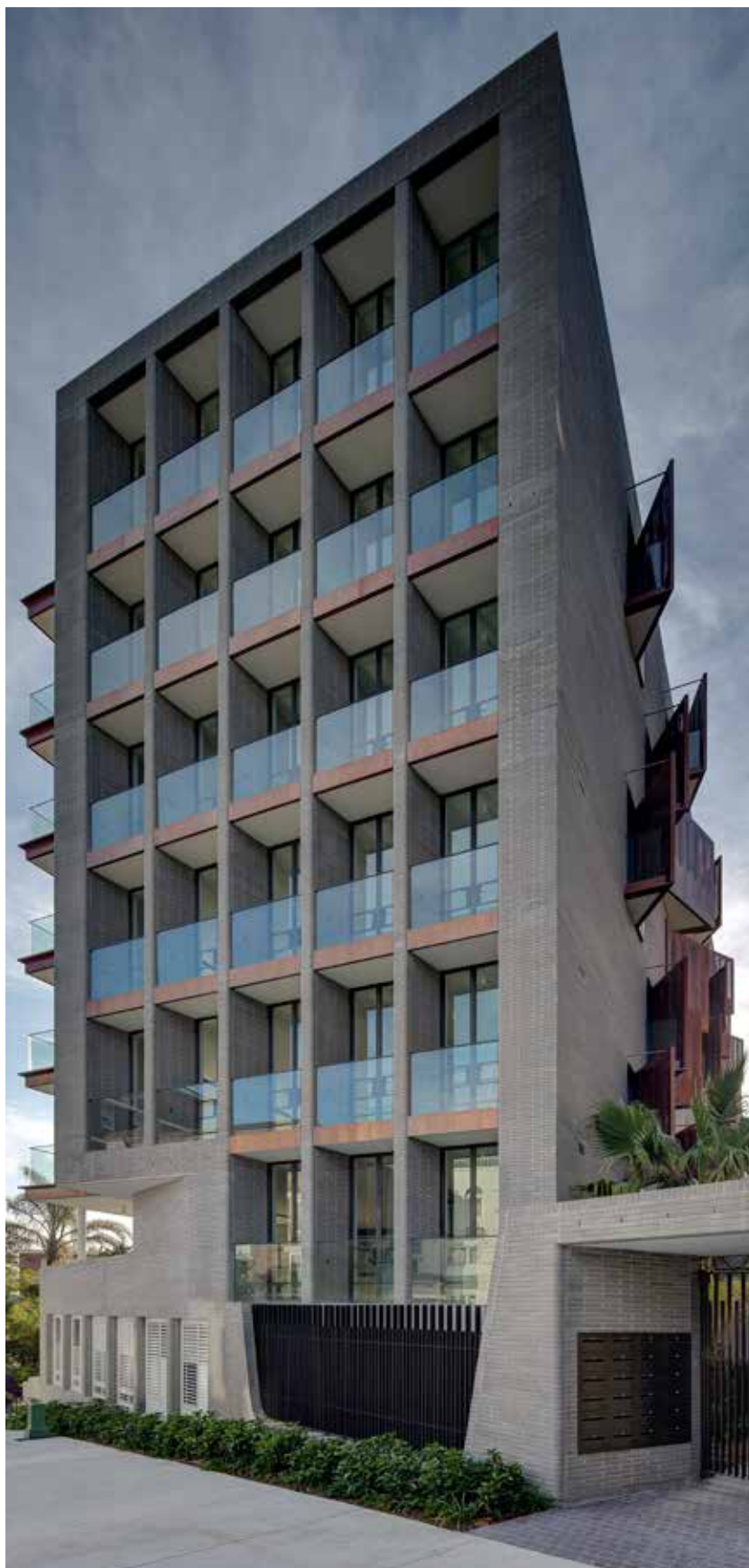
The west face of the completed project features colour-matched double-bullnose masonry units running the full height of the columns
