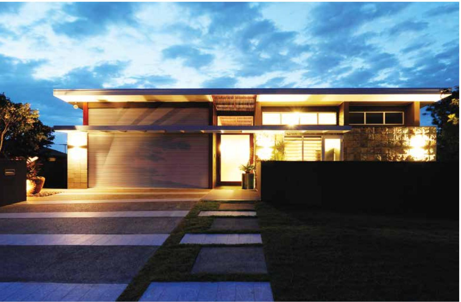
The distinctive triple-skillion roof form allows natural light to penetrate the interior through a central void. High- and low-level louvre windows open to capture prevailing breezes, enhancing cross-ventilation. Broad overhangs also block the worst of the summer sun while allowing the lower winter sun to penetrate and warm the interior.
