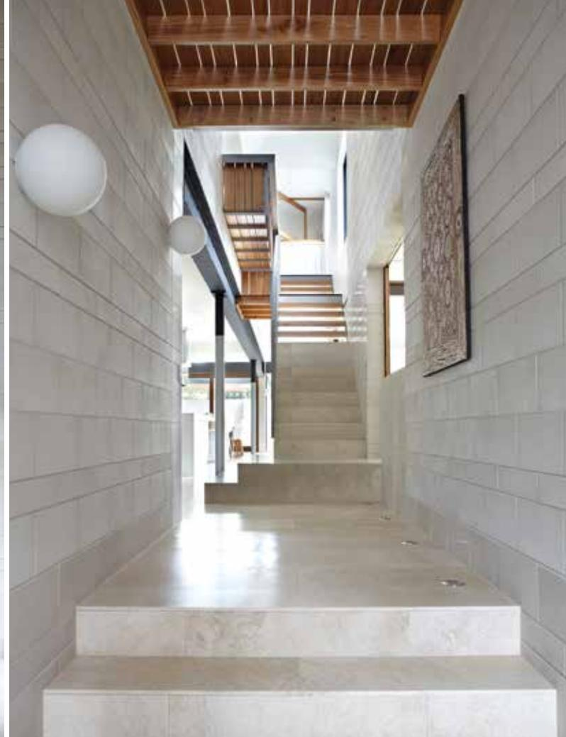
This substantial family home is built on a slab with a structure of four major masonry walls, one on each side boundary and two in the centre forming the circulation space. The blockwork walls are core-filled with steel reinforcement and concrete enabling them to be loadbearing and carry the structural loads such as the upper level timber flooring and roof structure.
