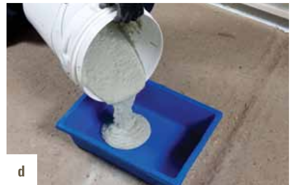
Figure 5: Mixing of Q Block Adhesive
