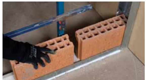
Figure 8: Q Block positioned and slid into place
