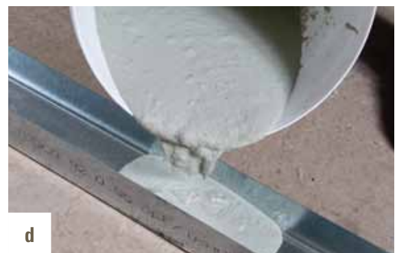
Figure 3: Installation of the tracks (a, b & c) and pouring self-levelling compound (d).
